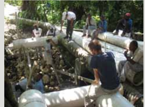
CEDC students and Haitians route pipe.
