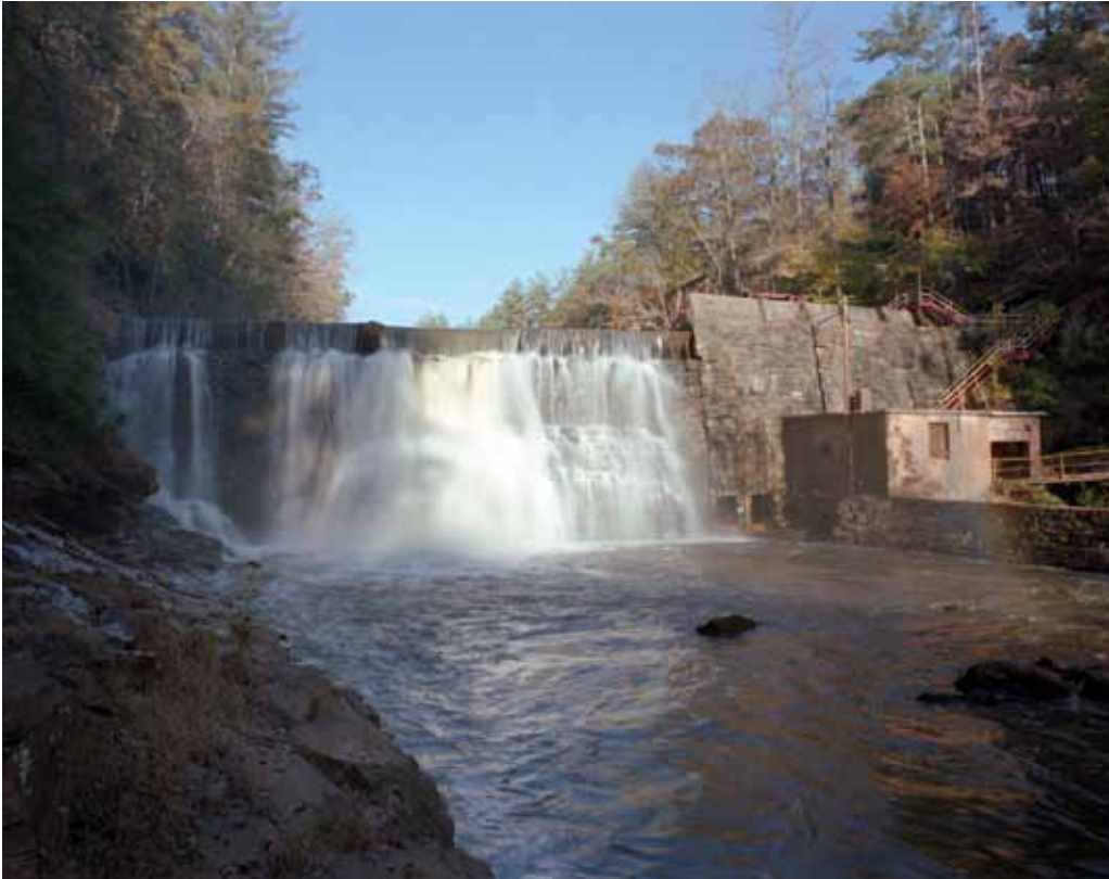
Woodside II Dam, Twelve Mile River, Pickens County, S.C. The dam was demolished in 2011 to remediate PCB pollution.
