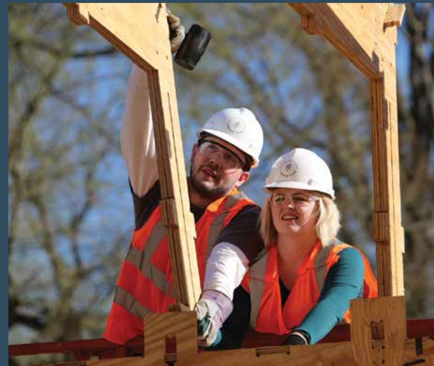
Justin Hamrick lugs a precut section of frame that has been numbered by the CNC machine—a computer-guided router—with its exact place in the structure. Hamrick has put several thousand miles on his truck driving back and forth to suppliers.
